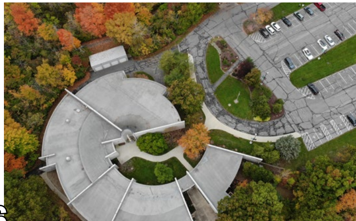
Aerial view of French Creek Nature Center
